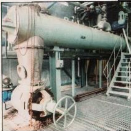
▲ Pre heater floor
